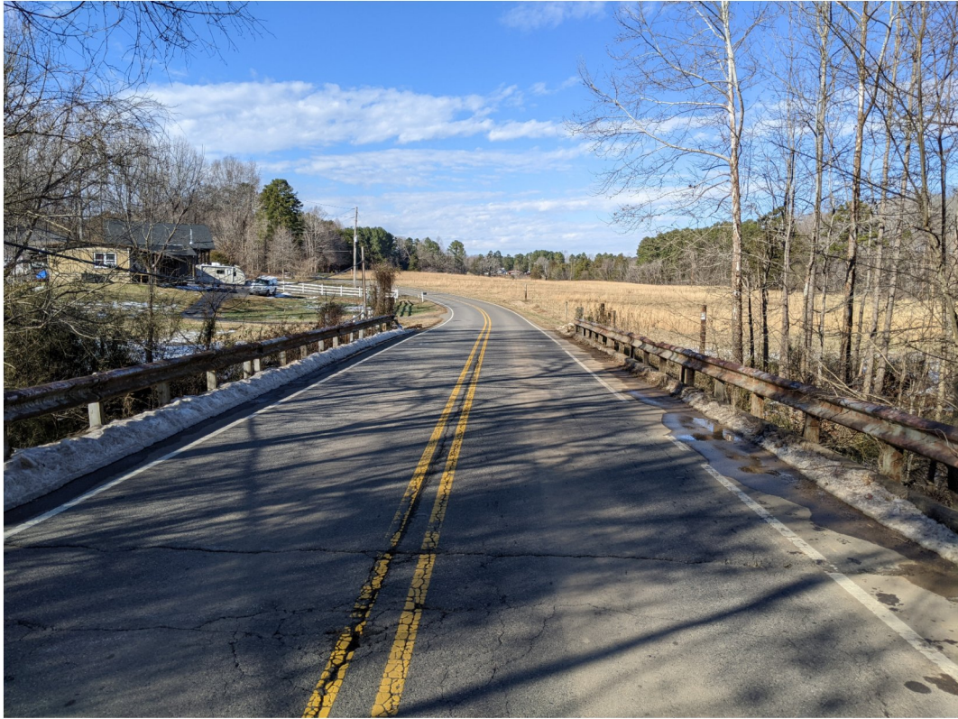
PHOTO 3 - VIEW UPSTATION FROM END BENT I.
